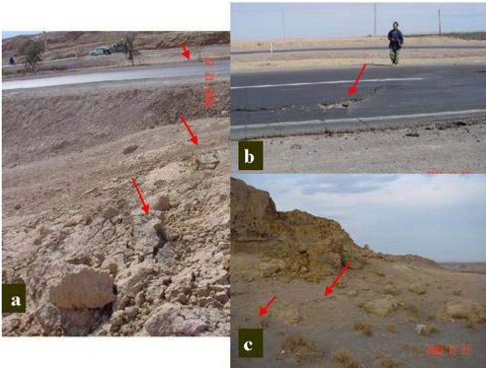
Figure-4: The surface fissures along the Bam fault (near Baravat) in the prone area of the 26/12/2003 earthquake). a) The fissures nearby Baravat, b) the fissure that ruptured the road from Bam to Baravat, and c) the fissures in the foot of the fault scarp of the Bam fault.
