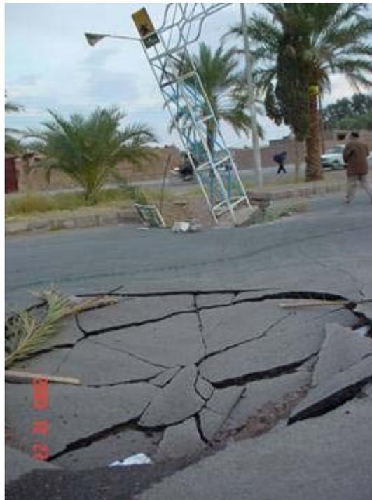
Figure-5: The sinkholes created during the 26/12/2006 earthquake in Baravat.
