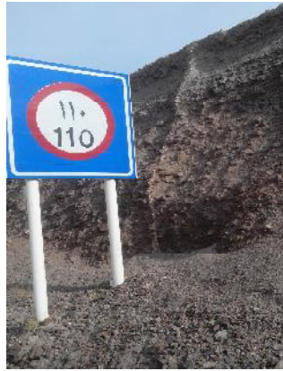
Figure 1. A photo of Robotkarim Fault in trench of Road (see toward east)
