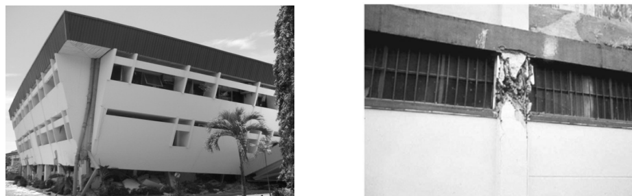
Figure 1. Negative effects of infill within structure; soft storey mechanism, Kusumastuti (2009) (left), short column mechanism Guevara and García (2012) (right)
