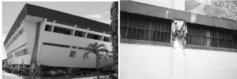
Figure 1. Negative effects of infill within structure; soft storey mechanism, (Kusumastuti 2010)(left), short column mechanism (Guevara and García)(right)
