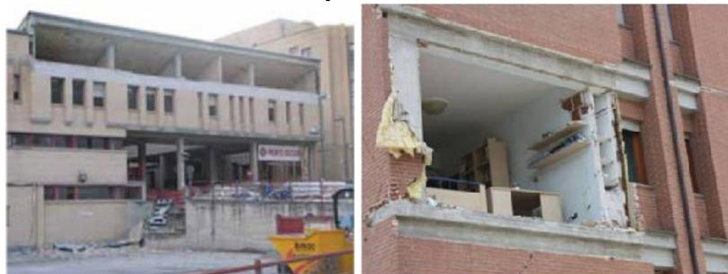
Figure 2. Damage in non-structural elements (Braga, Manfredi et al. 2011)
