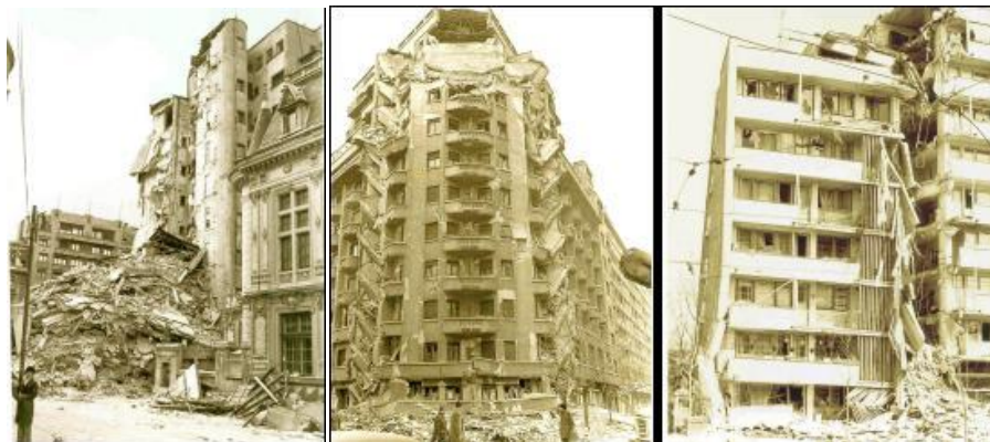
Figure 4. Total and partial collapse of the Bucharest RC tall buildings in 1977 earthquake
