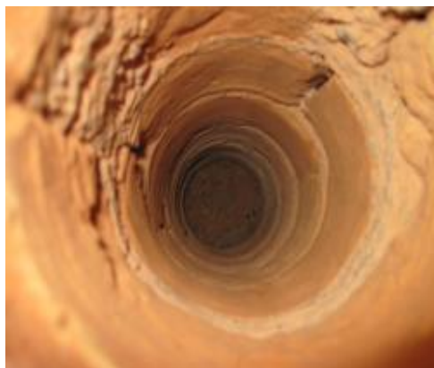
Figure 2. A vertical bore hole in a brick wall
