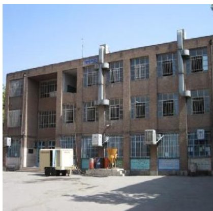
Figure 3. View of the selected building
