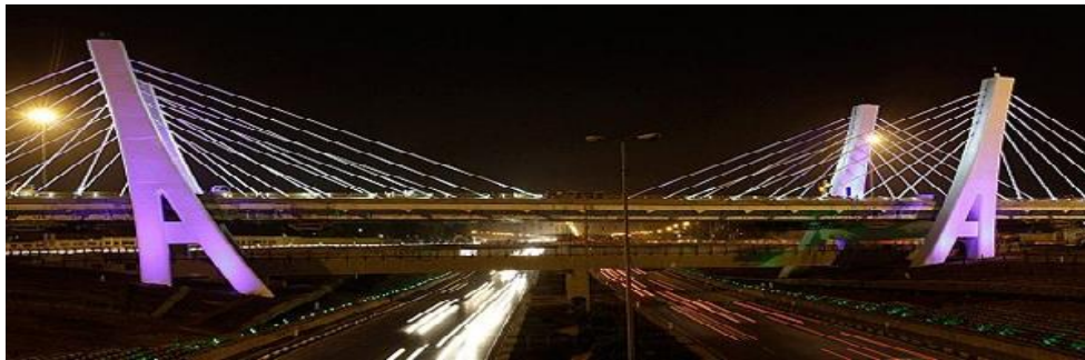
Figure 1. View of Mashhad cable-stayed bridge
