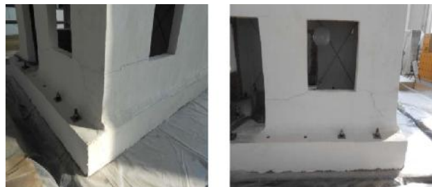
Damages on SismaCalce retrofitted model (1,22 g)
