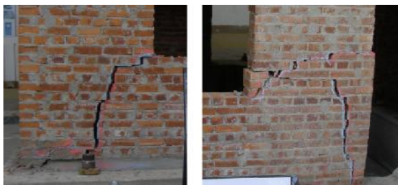
Damages on non-retrofitted model (0,35 g)
