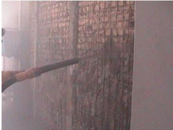
Figure 1. Adding Shotcrete layer to masonry wall
