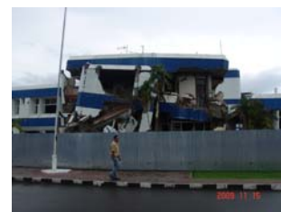
Collapse of the building, M Jamil Hospital
