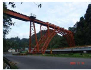
Railroad bridge on the way from Pariraman to Padang
