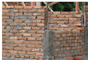
Lack of correct practice in masonry buildings
