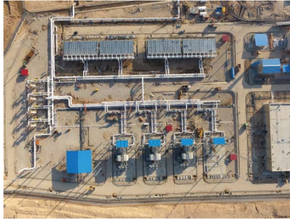
Figure 1. View of soil stabilized site with approximate 5 m jet grouting columns.
