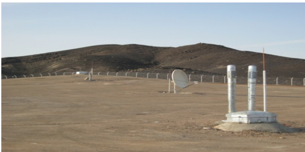
Figure 1. A new underground seismic station designed and constructed by IIEES.
