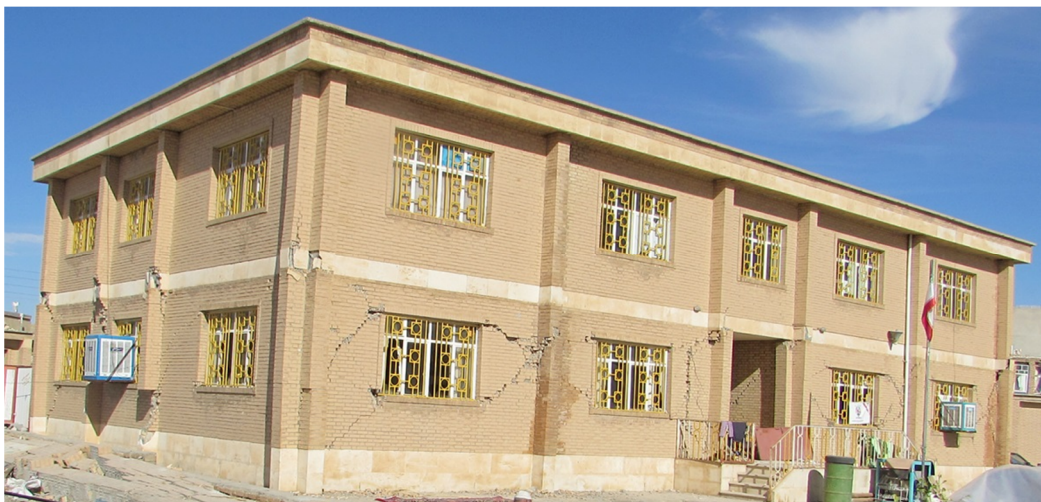
Figure 1. Damaged masonry building of Estesnaie School in Sarpol-e Zahab city in Ezgeleh Kermanshah earthquake.
