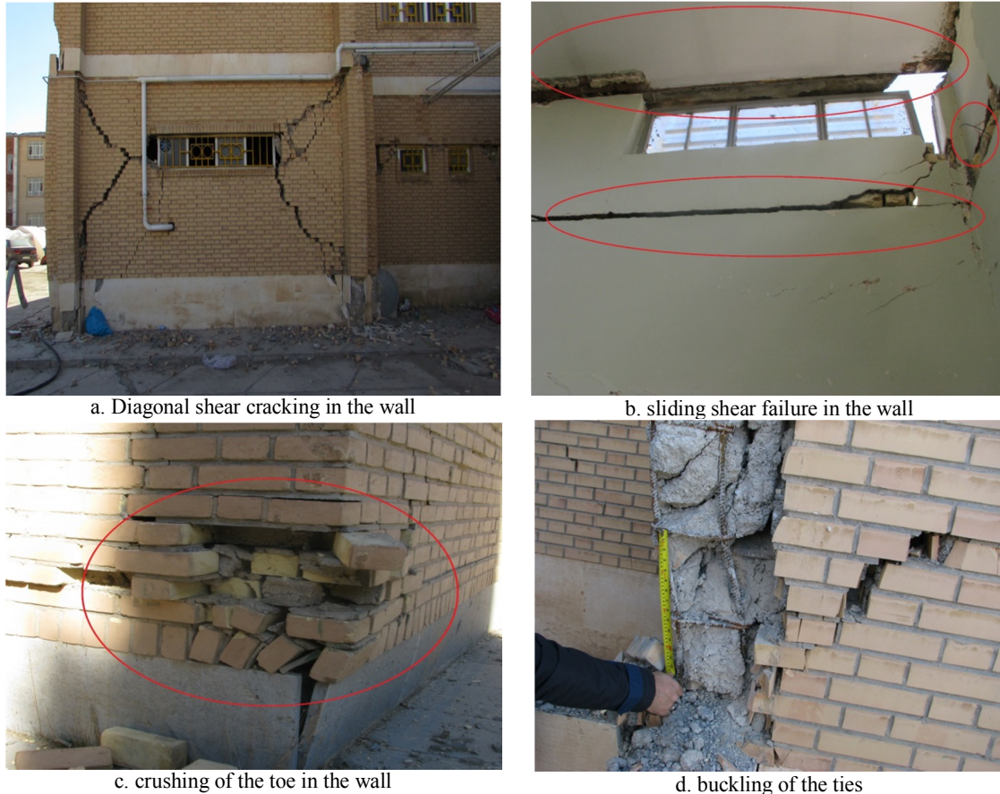
Figure 2. Different damage modes in masonry building.
