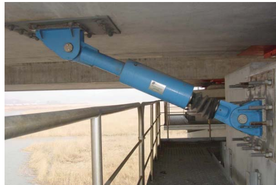
Figure 1. Force vs. Stoke behavior of FVD (Left Side), an installed FVD in a bridge (Road Co., 2017).
