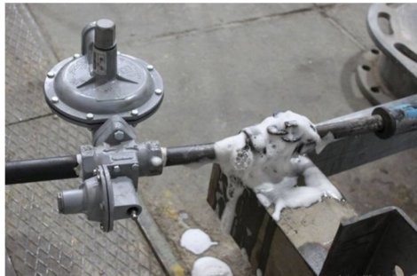
Figure 1. Failure process of the riser under lateral displacement.
