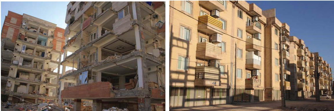
Figure 2. Site effects on two similar building complexes in Sarpol-e Zahab.
