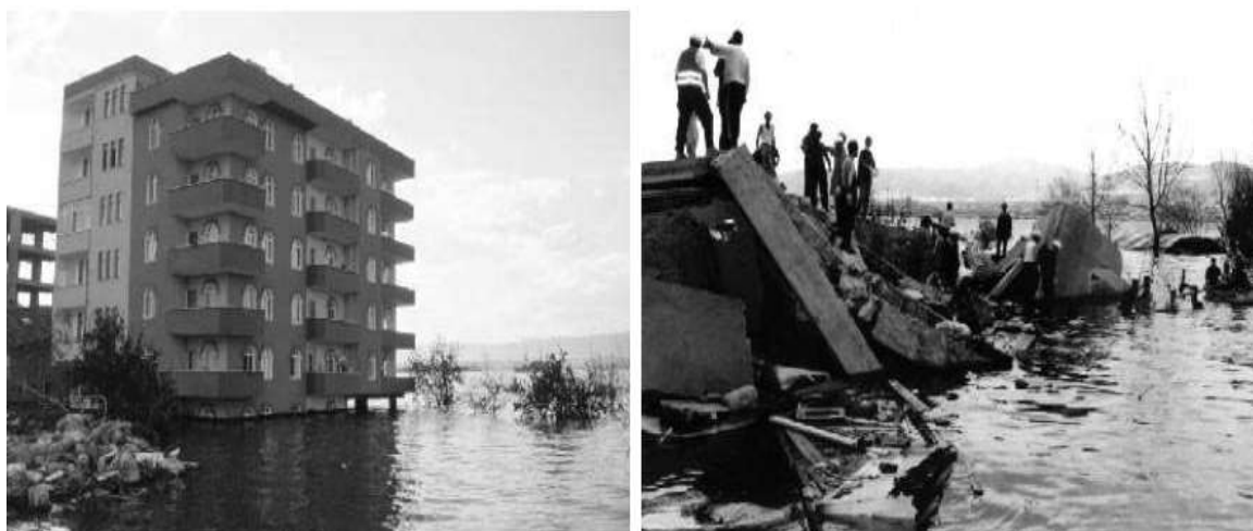
Figure 1. Collapse of a building caused by aftershock in turkey 1999 (Yeo & Cornell, 2005).
