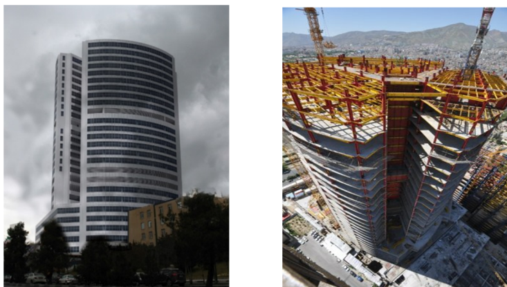
Figure 1. (left) Schematic 3D view of the building, and (right) a photo of constructed structure.
