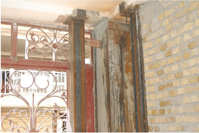
Figure 3. columns strengthening by steel Jacketing.
