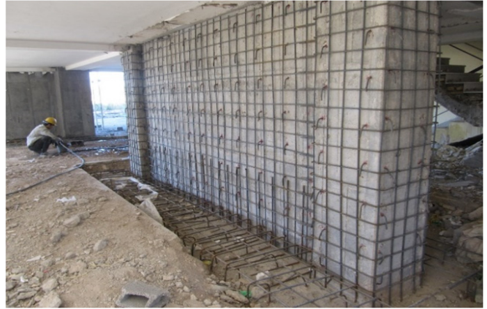
Figure 4. Meshing on the shear wall.
