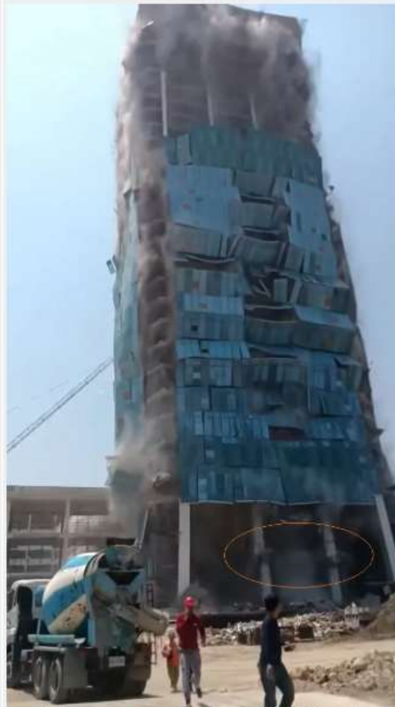
Bangkok Tower: Notice the shearing off of the columns
